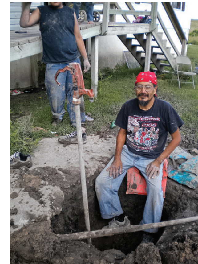
A local Pine River Reservation resident works on a pump to provide a house with well water.
